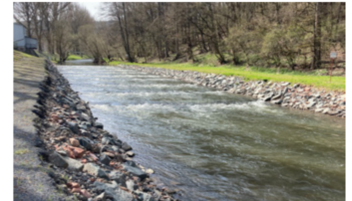
Today there are several natural stone bars for the fish to overcome
