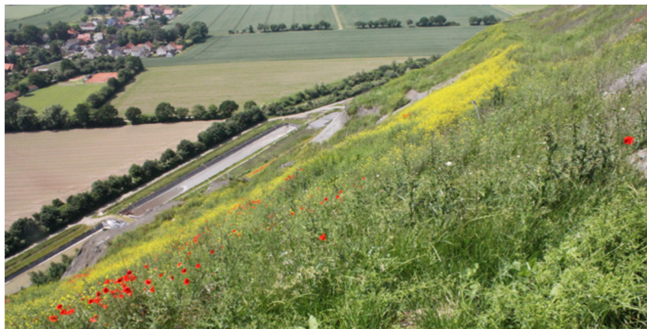
A tailings pile greening system absorbs rainwater and reduces the formation of saline tailings pile water
