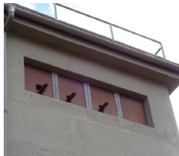
A former border tower is home to nesting sites
