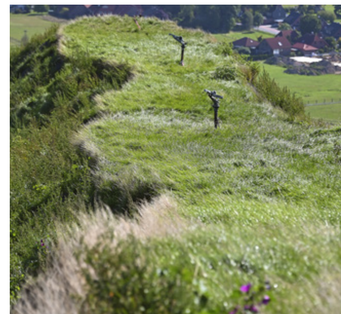
In the start-up phase, the greening is irrigated, as here on the tailings pile top
