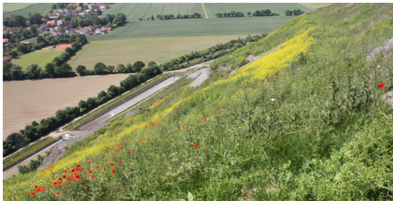
A tailings pile greening system absorbs rainwater and reduces the formation of saline tailings pile water
