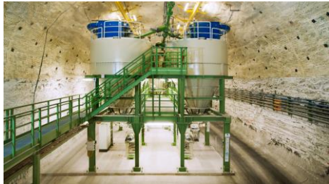
Thick matter backfill
