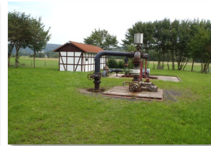
Deep well injection (for K+S in the Hessian-Thuringian potash district until the year 2021)
