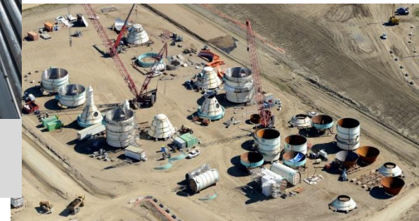
Pre-assembly vessels ECC started (on site)
