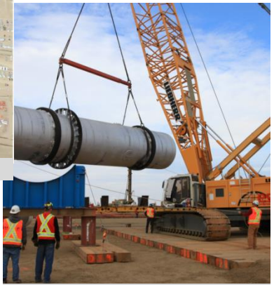
Off-load drum dryer at Legacy site
